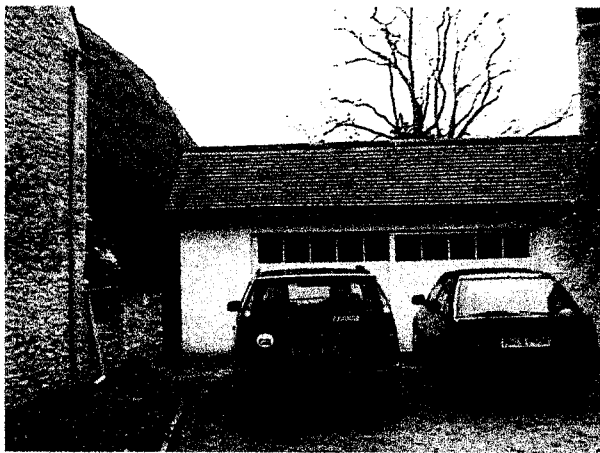
Garage Front (North)
